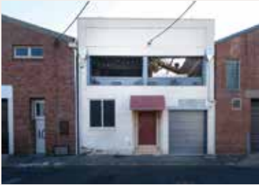
Power House CKDS Architecture Residential Architecture - Houses (Alterations and Additions)
